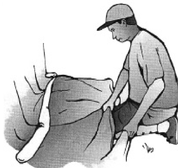
Figure 5.5 Using snakes to ensure a good ground seal
